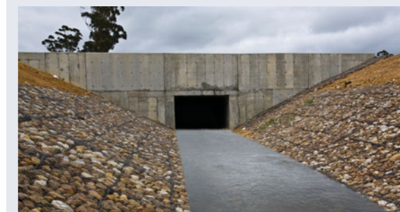
ABOVE Stormwater channel, Drommedaris, Drakenstein (2009): The project consists of the construction of a 1:50 year flood catchment channel for the Berg River that is situated between Paarl and Worcester which is the main feed to surrounding wine farms and vineyards. The construction of the channel was necessary in order to prevent the flooding of the Mbekweni Township as well as the new Drommedaris Development during rainy seasons. CSM Project Management, Civil Engineering and Construction Monitoring Divisions were involved in the project
